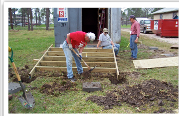
Work Projects Together
